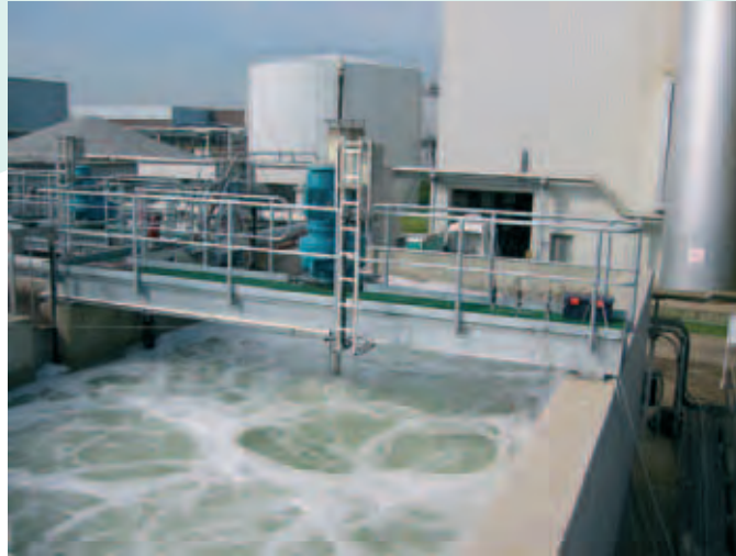
1 out of 9 HYPER-CLASSIC® -Mixer/Aerators in an industrial wwtp in Belgium (Pulp & Paper Industry)
