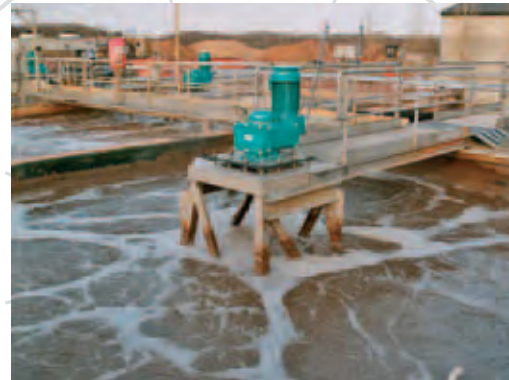
4 HYPER-CLASSIC ® Mixing & Aeration Systems in an industrial wvtp in Belgium (Food Industry)
